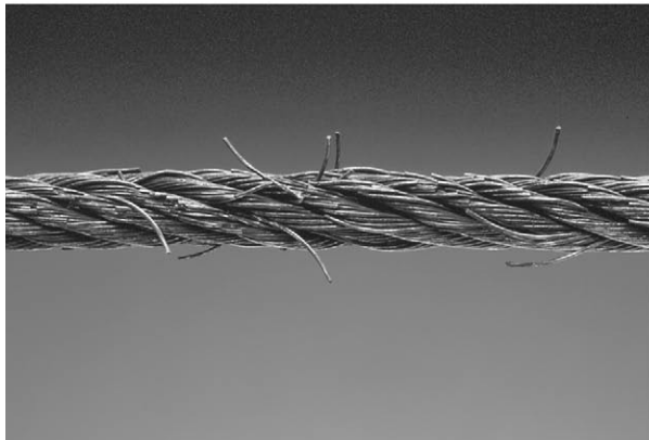
Cable With Severe Corrosion
